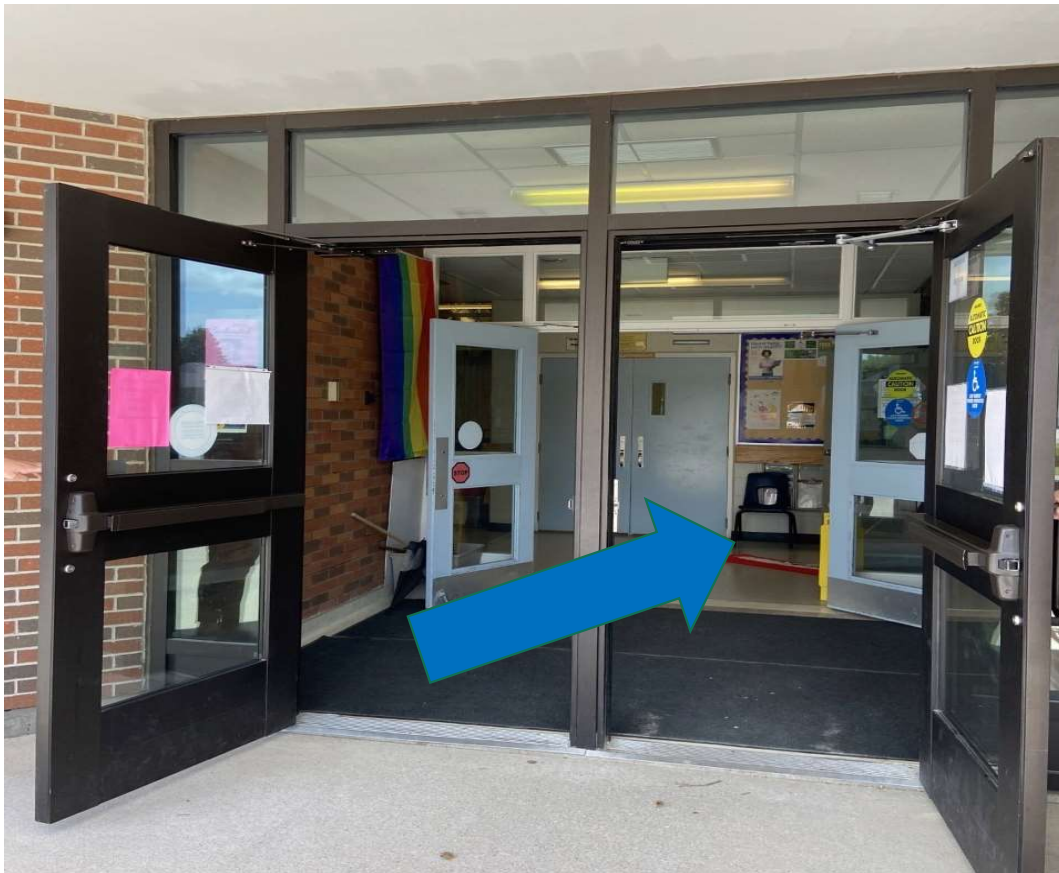
Main Entry – Front Doors
